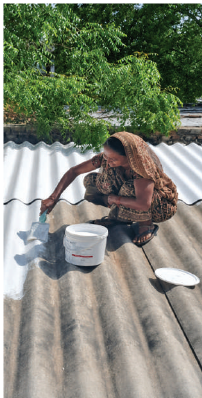
A resident of Bhattiwada in Patan applies white solar reflective index paint to the roof of her house to cool it
