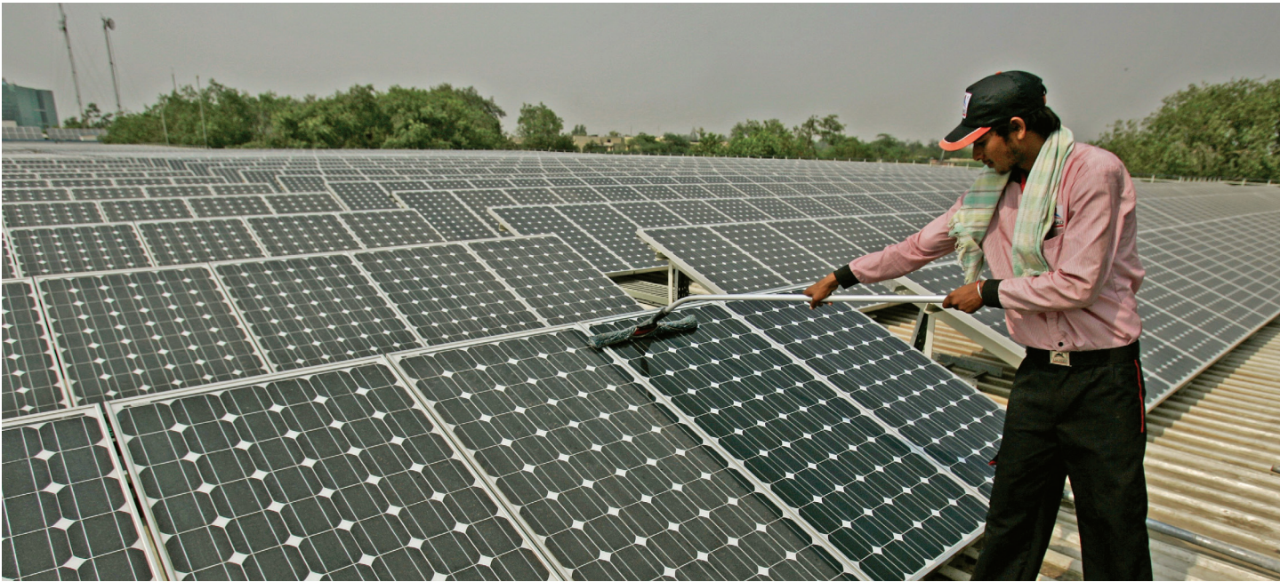
A solar panel being cleaned at a site near New Delhi
